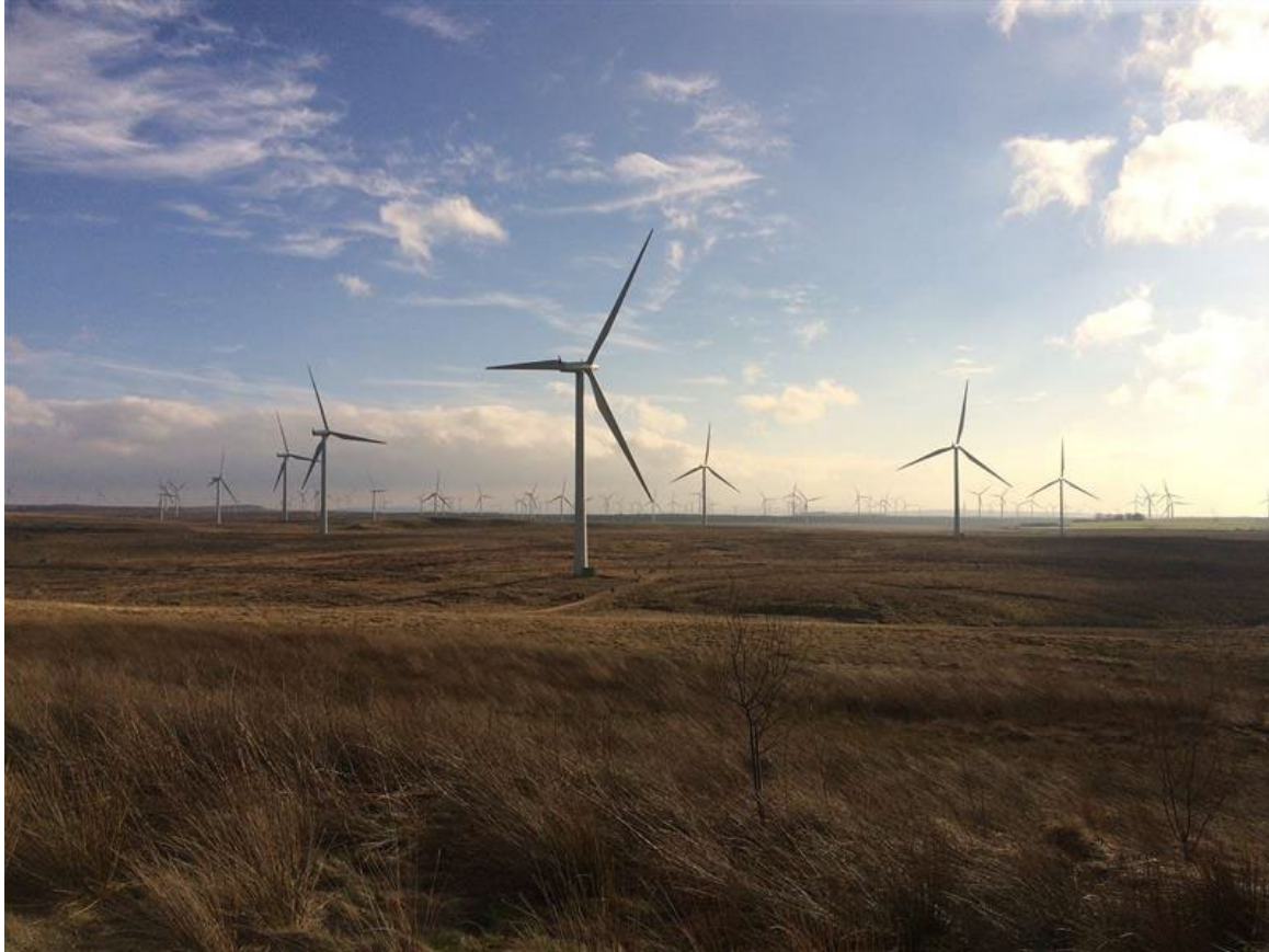
Figure 2: Photo of Whitelees near Glasgow. Largest land-based windfarm in Europe, where power costs are 4x just 200m down the road.
